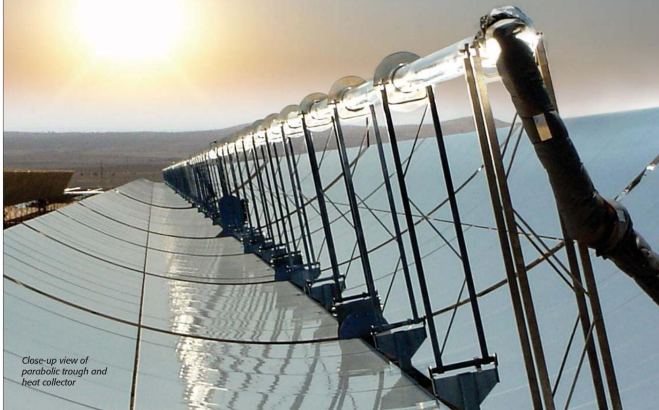
Close-up view of parabolic trough and heat collector
