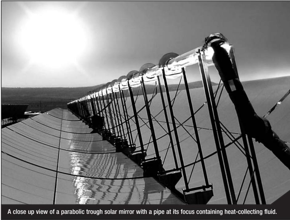
A close up view of a parabolic trough solar mirror with a pipe at its focus containing heat-collecting fluid.
