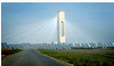
**Feed into the grid cheap, reliable energy from solar thermal power stations** in the sun-rich areas of Southern Europe, North Africa and the Middle East. These power stations, like this one in Spain, use mirrors to concentrate the sun's heat to boil water and drive a steam turbine.
